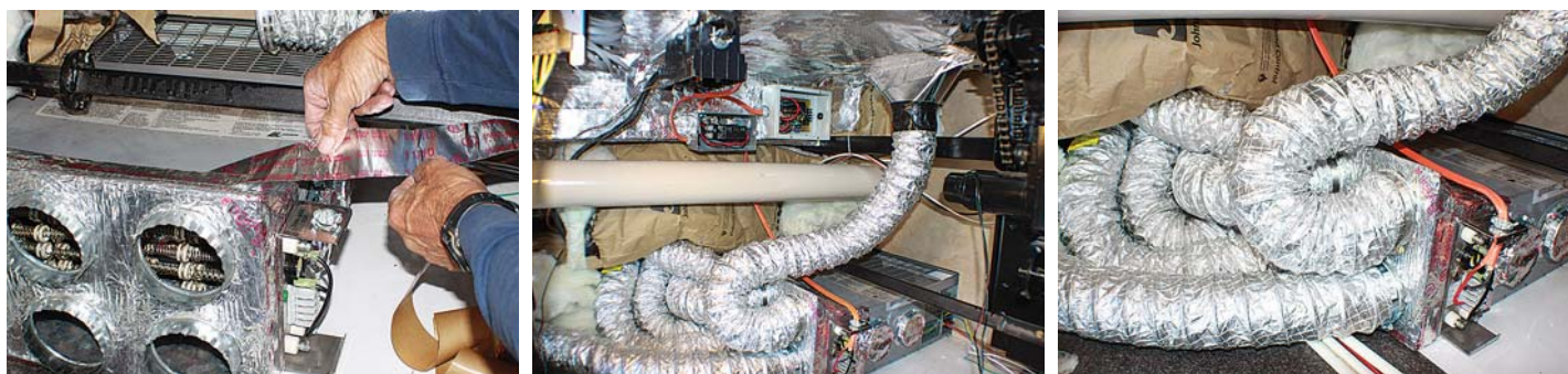
(Below, from left to right) After the heating element is installed into the plenum, the plenum is installed to the rear of the furnace and high-temperature aluminum foil tape is used to seal the edges. At the top the junction box for the 50-amp service is installed. Below is the disconnect switch, and to the right the system controller is mounted. The orange, 10-gauge Romex runs between the J-Box to the disconnect switch to the controller then runs down to the heating element. The flexible heat ducting is attached to the plenum.
