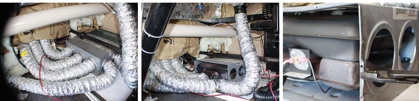
(Above, from left to right) Flexible ducting is routed from six ports in the stock Suburban furnace in the test fifth-wheel. The ducting and collars are removed from the rear panel of the furnace to start the installation process. On this Suburban furnace, pliers were used to fold the tabs flat on both sides of the furnace to allow the new plenum to fit properly.
